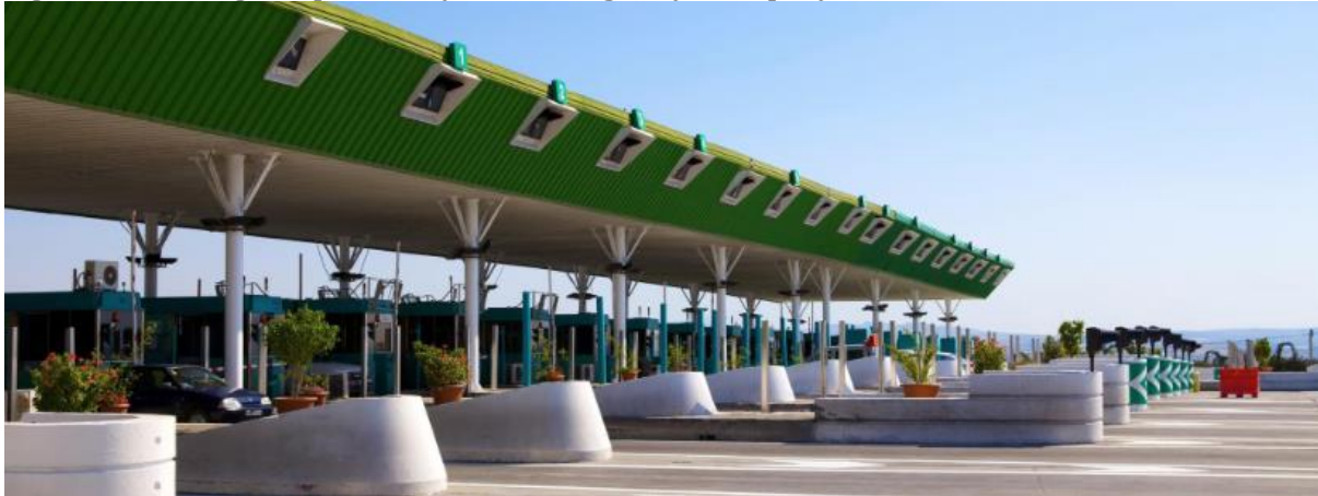
Figure 3-51: Toll gate operated by Tunisia Highways Company
