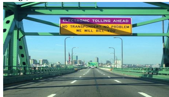
Figure 2-29: Electronic tolling system on Tobin Bridge, Massachusetts
