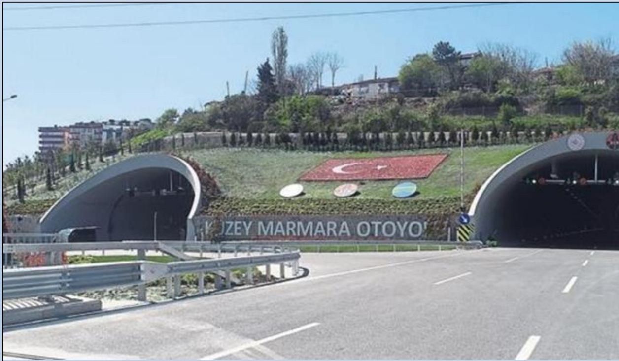
VMS in Northern Marmara Motorway Tunnel
