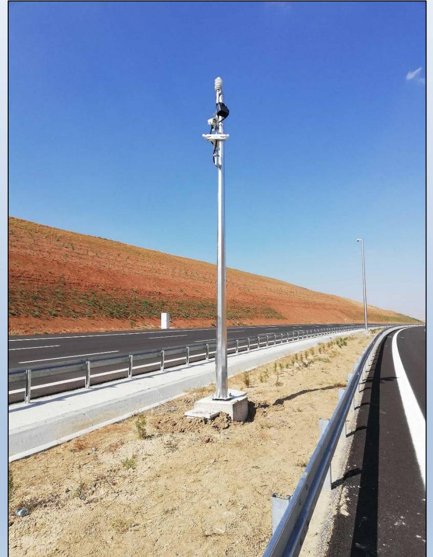
Meteorology Station in Ankara-Niğde Motorway
