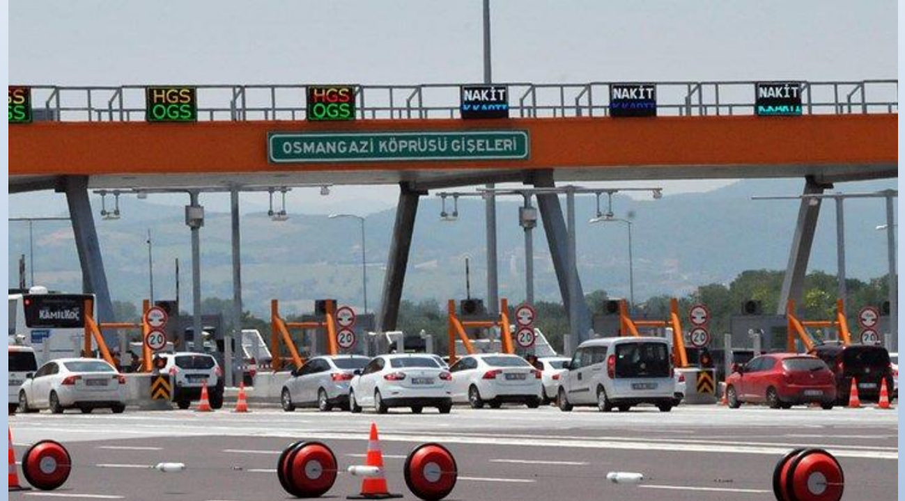
ETCS gate in Osmangazi Bridge
