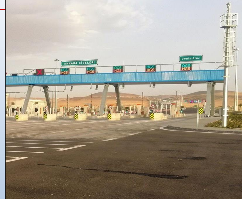
ETCS Gate in Ankara-Niğde Motorway
