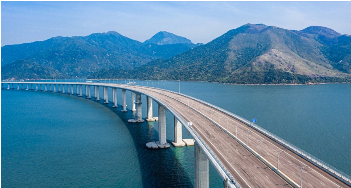
Figure 26 Hong Kong–Zhuhai–Macao Bridge (HZMB), China
