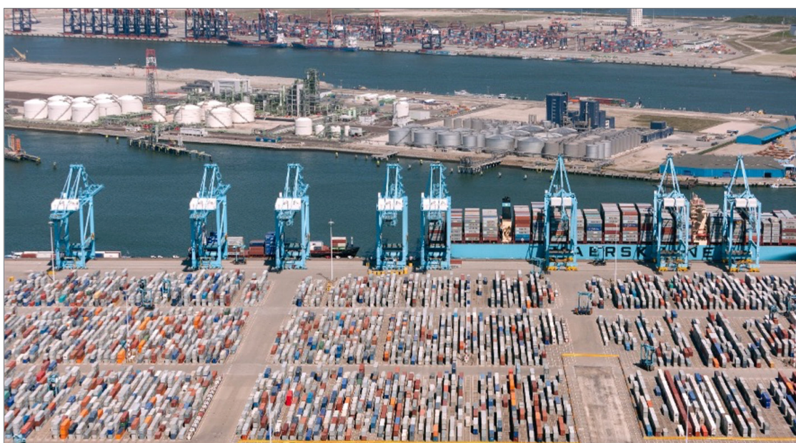
Figure 32 Port of Rotterdam, The Netherlands
